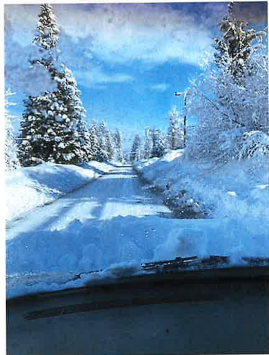
Without shoulders, Davis Ave travel lanes get very narrow in winter.
